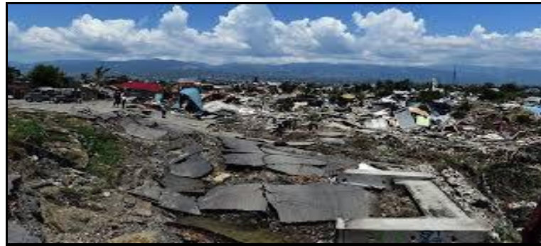
Figure 5.2 Soil liquefaction example
